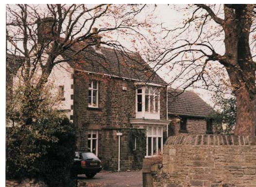
Cross Grove House at the top of Hillfoot Road
