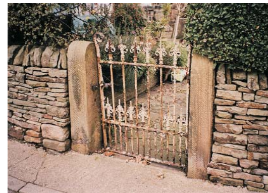
Old iron gate and stone wall, Totley Hall Lane
