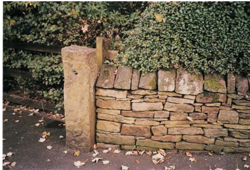
Characteristic stone wall with triangular coping
